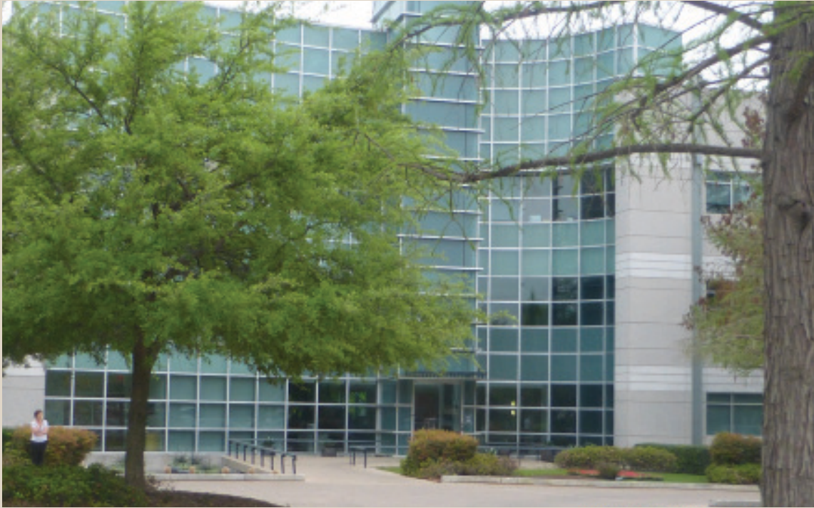
Westdale Royal Ln., LP located at 100 Royal Lane East.
